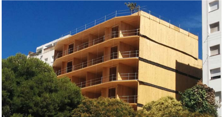
The La Borda Cooperative Housing Building, Barcelona. Made with CLT (cross laminated timber) pine. It is currently the tallest wooden building in Spain. Photo: INCAFUST, CTFC.
