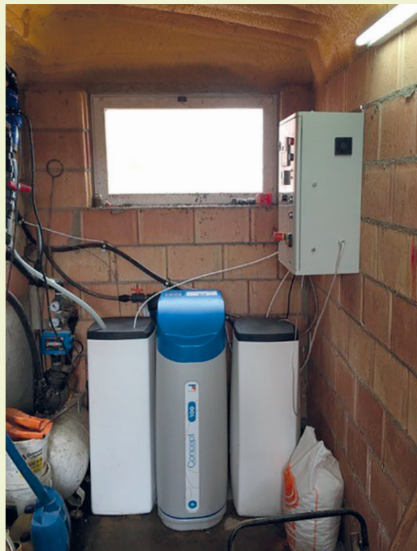
Figure 2. Installation of the electrolysed water unit at the fattening farm. Photograph: Xavier Puigvert.
